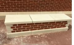
Cast stone features are: veneers, cornerstones, wall capping, benches, and pavers.
